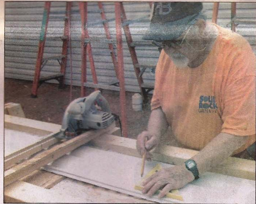
Volunteer Jack Hedrich of Park Ridge, Ill., marks a line to cut siding.
